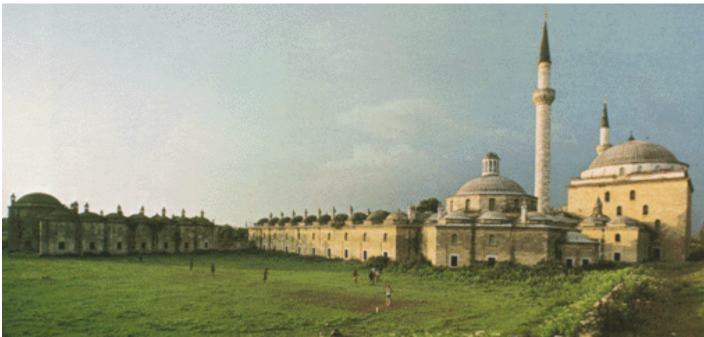
General view of Bayazid II Kulliye
